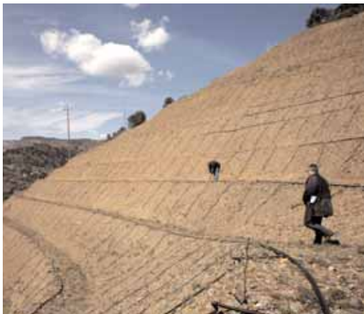
Natural land with a gradient of over 60%. The slopes do not exceed 2 m in height; slope plantation
