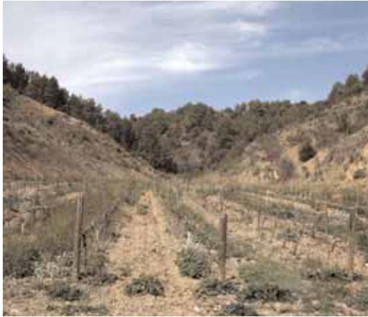
Vineyard built by filling in a natural gully instead of forming terraces on the mountain with drainage to the gully
