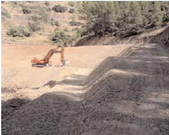
Terraces with a constant lengthways gradient and width
