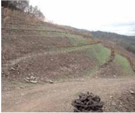
Plant cover being formed
