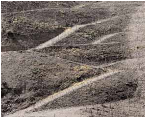
Zigzagged accesses to terraces to improve occupational safety
