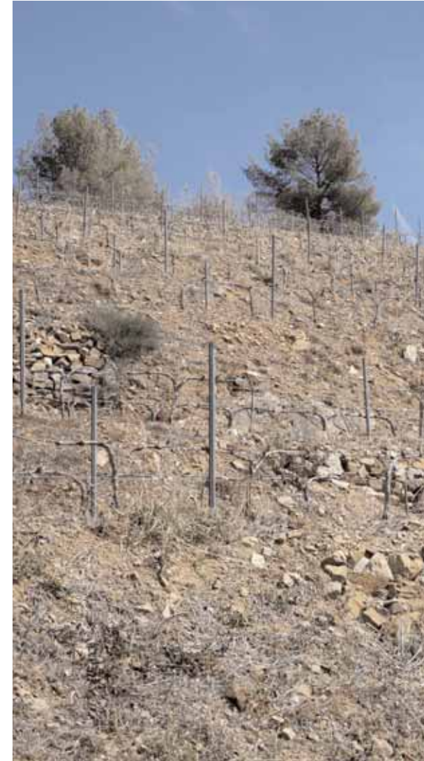
Repairs on eroded slopes
