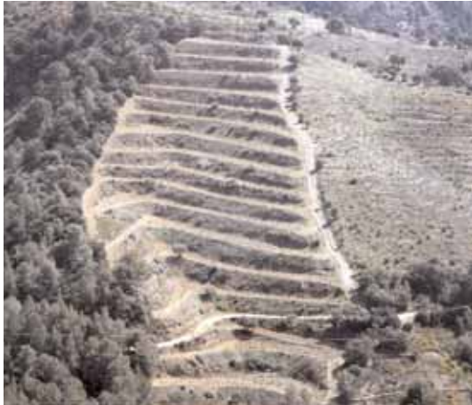
Occupational risk: perpendicular accesses to level lines with an excessively steep gradient
