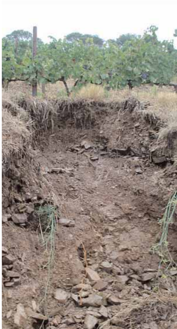
Severe erosion on a slope, putting some stock at risk
