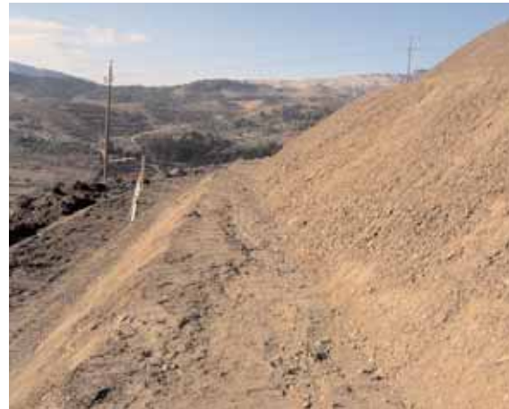
Slope finishing with a constant height by laser levelling
